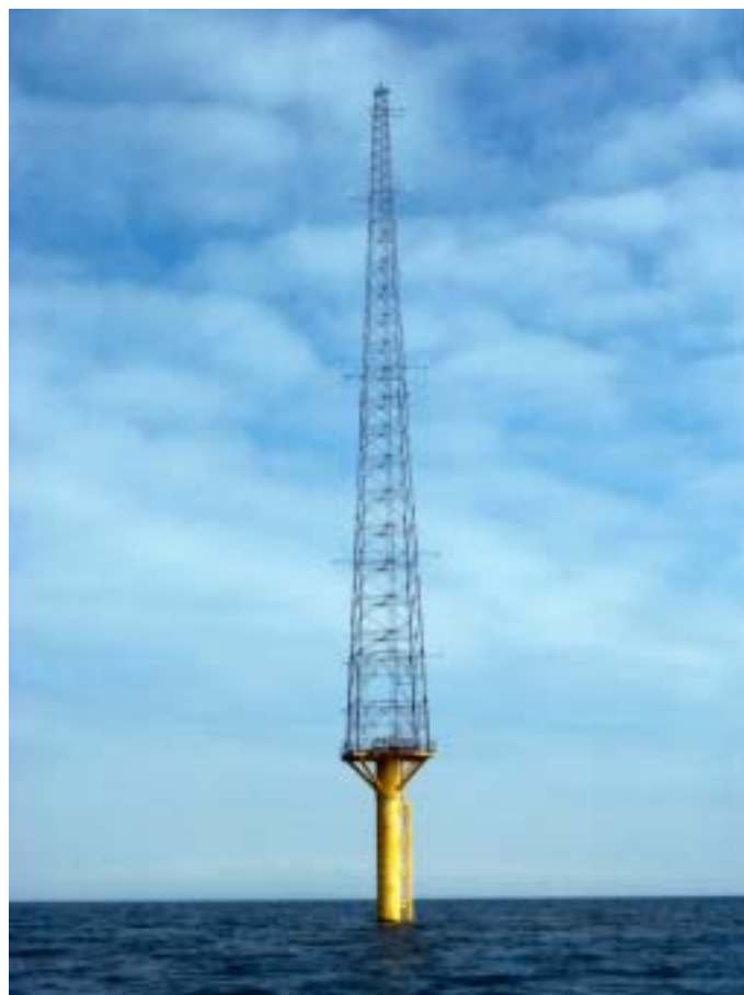
Meteorological mast, Morecambe Bay, UK: instrumented for wind measurements at five heights prior to design of the Shell Flats wind farm
